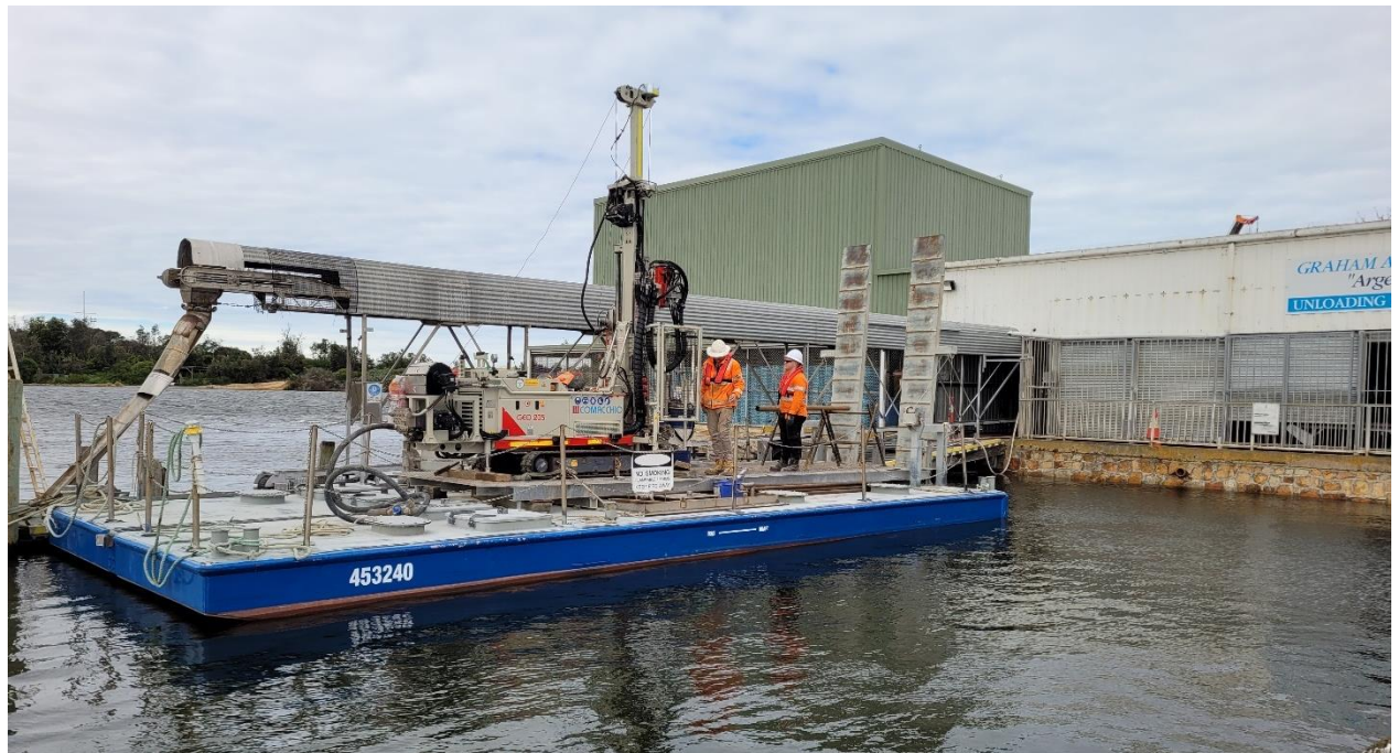
Image 3 - View of the drill rig setting up on the barge.
